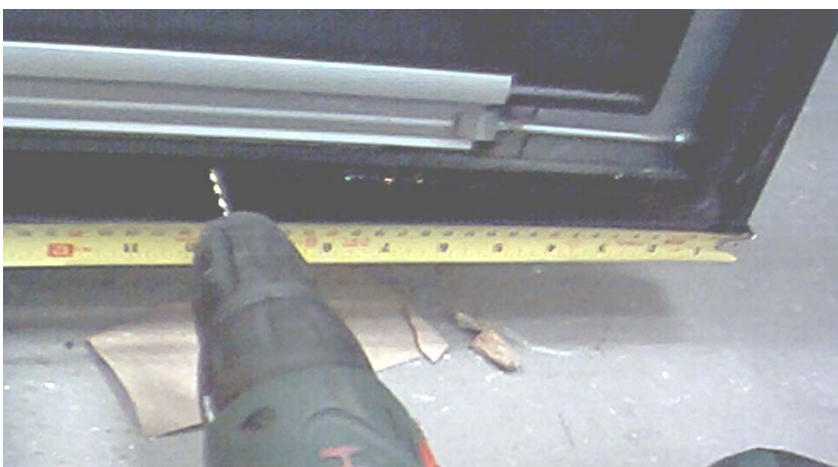
Figure 4.6.2. Drilling first hole in Door
