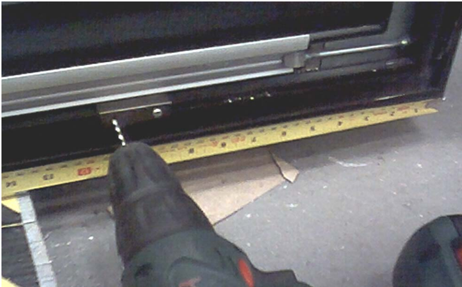
Figure 4.6.5. Drilling out second hole
