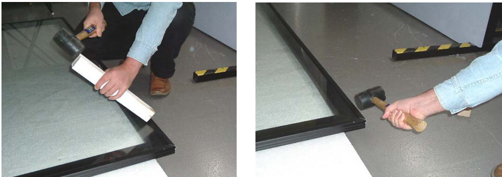
Fig. 4.2.4. Glazing Retainer Removal and Replacement
